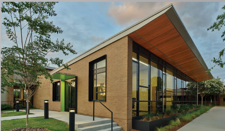
PROJECT: ROCK REGION METRO HEADQUARTERS ADDITION FIRM: AMR ARCHITECTS CONTRACTOR: BELL CONSTRUCTION CO. INC. LOCATION: NORTH LITTLE ROCK, AR
