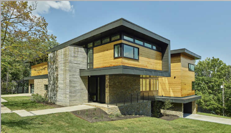
PROJECT: WOLFE RESIDENCE FIRM: DEMX ARCHITECTURE CONTRACTOR: GB GROUP CONSTRUCTION LOCATION: FAYETTEVILLE, AR
