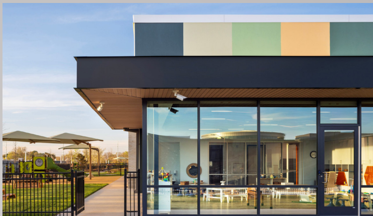
PROJECT: LITTLE SQUIGGLES CHILDREN'S ENRICHMENT CENTER FIRM: PAGE CONTRACTOR: CADDELL CONSTRUCTION LOCATION: BENTONVILLE, AR
