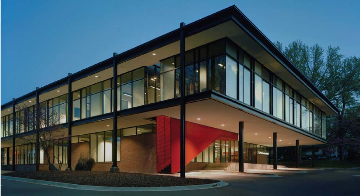
The Fulbright Building in Fayetteville.
