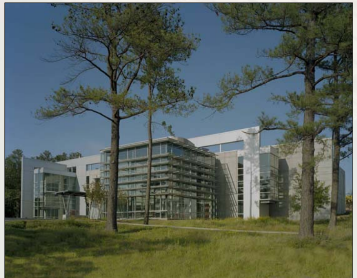
The 2007 Member Choice Award went to Polk Stanley for the Acxiom Central Arkansas Data Center (above).
