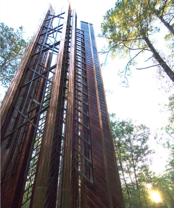
Anthony Trust Carillon Tower at Garvan Woodland Gardens.
