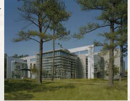
Acxiom Data Center
